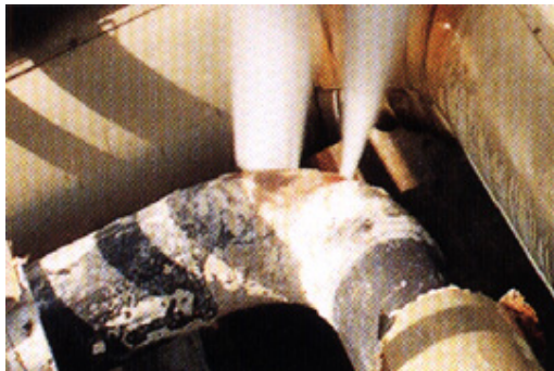
Piping System Leaks
