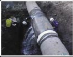
Repair of "Out of Round" Pipeline with Composites and Repair Sleeve
