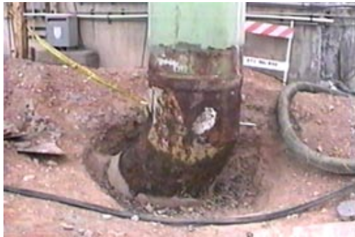
Corroded 4" Water Line
