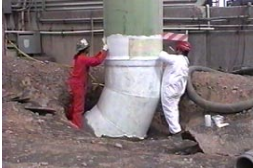
Repair of Corroded Water Line
