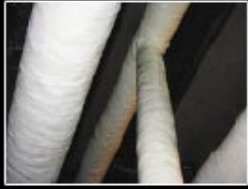
Repair of Corroded Service Pipe
