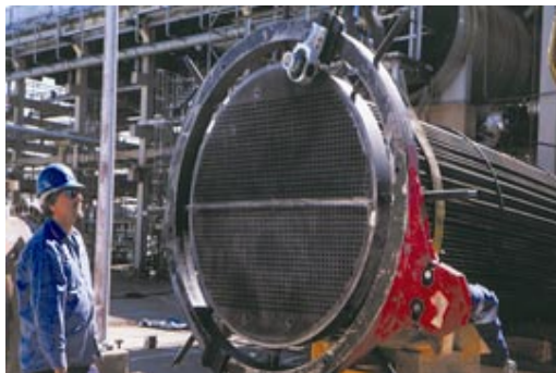
Re-machining gasket surface of tube sheet using OD mount flange facer
