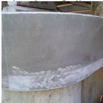
Composite repair of bridge support
