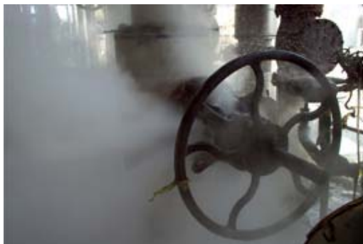
Before - Steam Leak on Valve Packing
