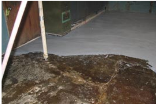
Concrete Overlays Before
