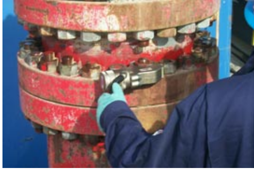
Assembling flanges with low clearance hydraulic torque wrench
