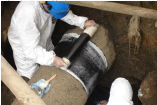
Repair of Dented Pipeline
