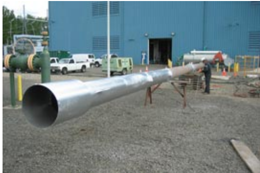
Cogen Stack After
