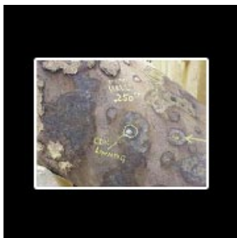
Repair of Corroded Service Pipe
