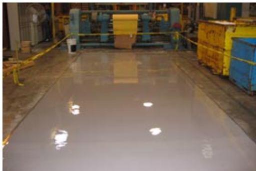
Chemical Resistant Flooring
