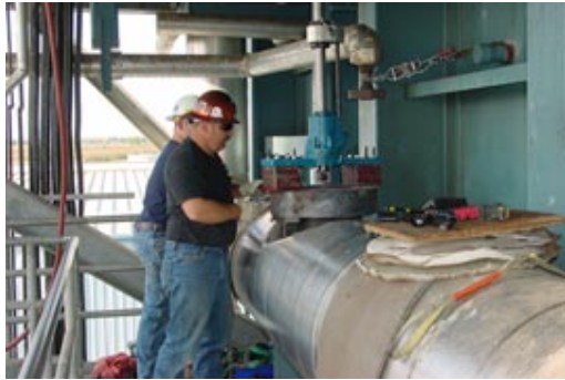
Boring header nozzle flange with 1" boring bar
