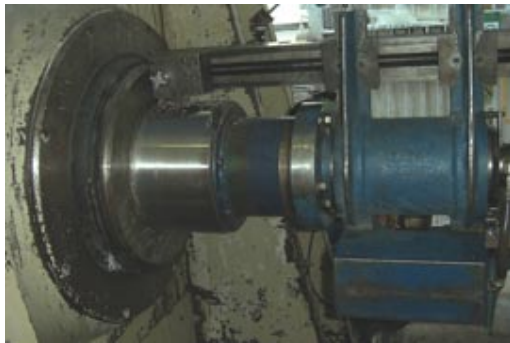
In place machining of shaft bearing surface
