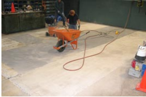
Concrete Overlays Before
