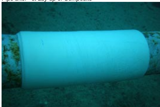
After 2nd Lay-up of Composite
