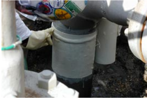
Repair Over Corroded Weld on Pipe
