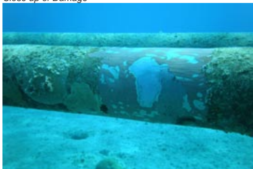
Cleaning the Dented Location
