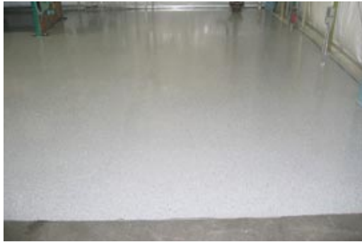
Crack Repair / Pressure Injection
