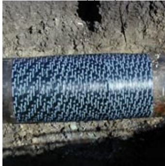
Dented and cracked pipe repaired with composite wrap
