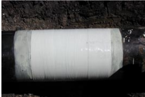
Dented Pipe repaired with Composites
