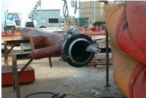
Counter bore & bevel on pipe spool using clamshell
