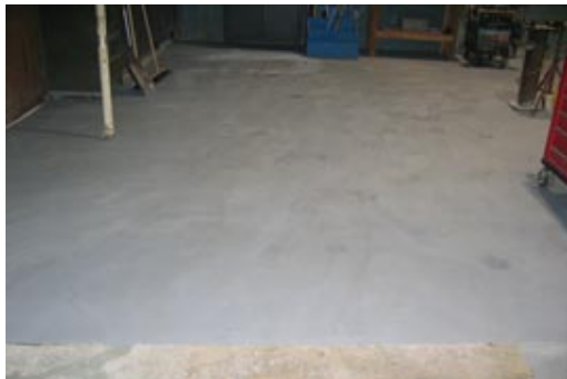
Concrete Overlays After
