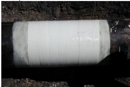
Repair of Pitted Pipe
