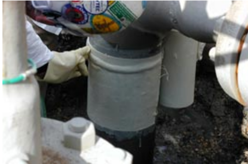
Repair of corroded 4" crude oil line over weld
