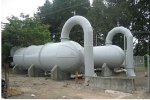
Sand Filters After
