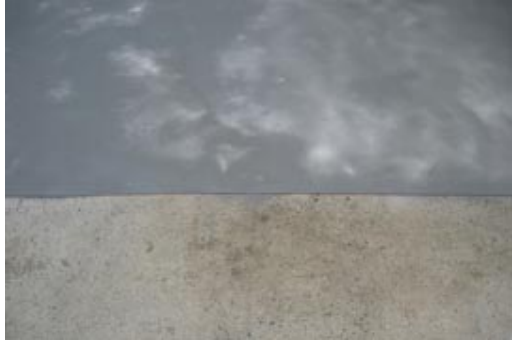
Concrete Sealing / Polishing
