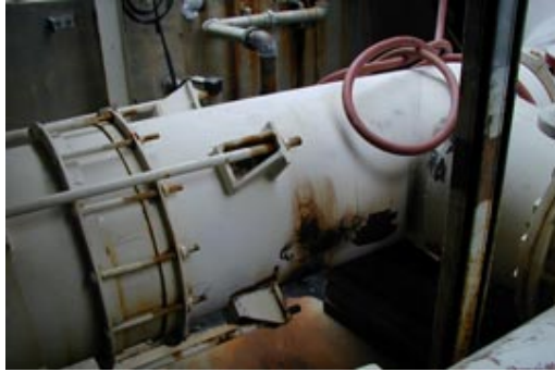
Corroded 14" effluent Water Line
