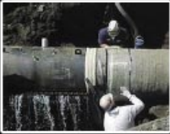
Repair of "Out of Round" Pipeline with Composites and Repair Sleeve
