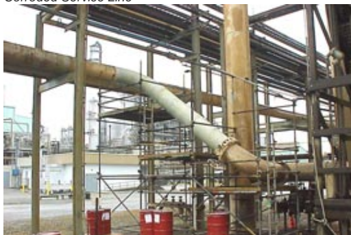
Repair of Corroded Pipe
