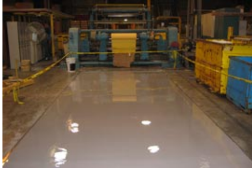
PM Winder Floor After
