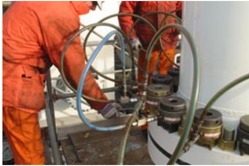
Assembling flanges using hydraulic tensioning equipment
