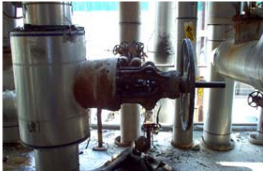
After - Repaired Steam Leak on Valve Packing
