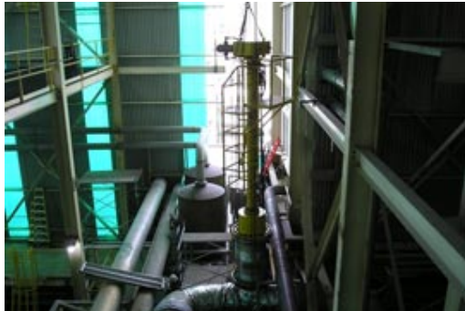
7 1/2" Hot Tap in Industrial Manufacturing Plant
