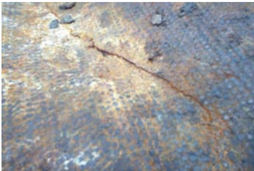
Dented and cracked pipe
