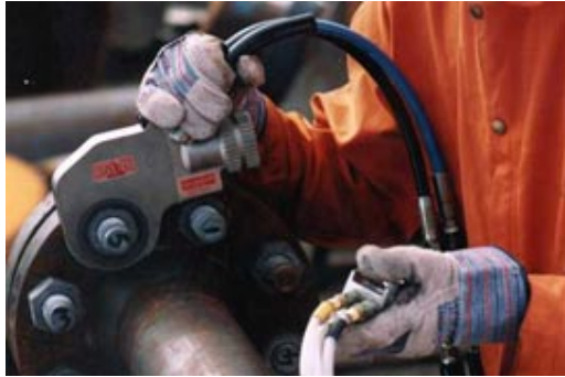
Assembling flanges using hydraulic torque wrench
