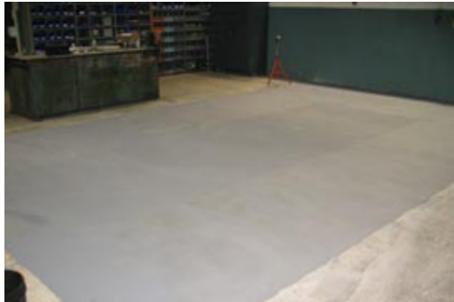
Concrete Overlays After
