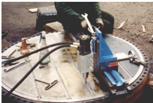
Milling of partition groove on exchanger dollar plate.
