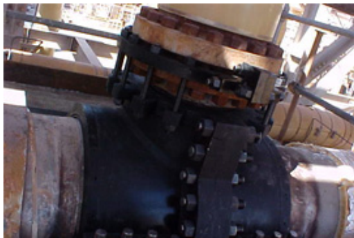
Custom Engineered Leak Repair Solutions
