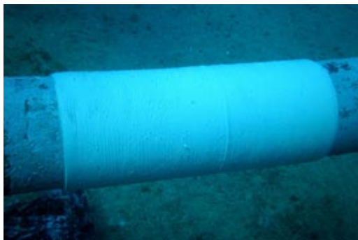
Pipe after 1st Lay-up of Composite
