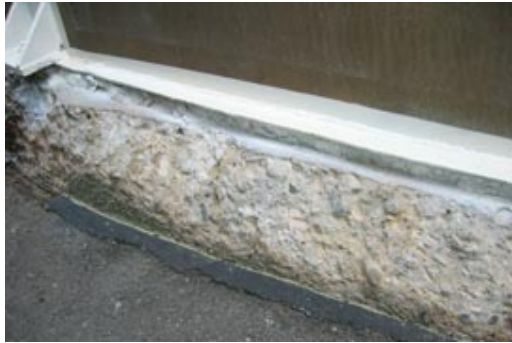
Tank Base Before
