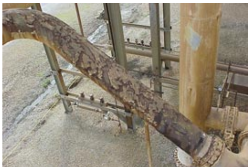
Corroded Service Line
