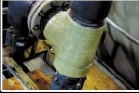
Repair of 4" Cracked Tee
