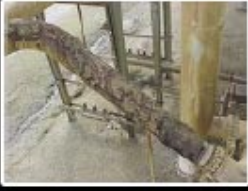
Repair of Corroded Service Pipe
