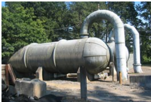
Sand Filters Before
