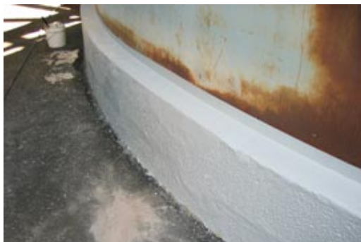
Tank Base After
