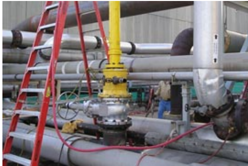
Hot Tap in Manufacturing Plant
