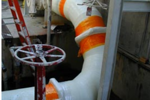
Corroded 14" effluent Water Line Repaired with composites
