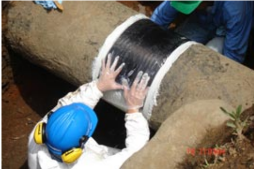
Repair of Dented Pipeline
