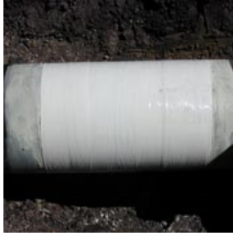
Dented and cracked pipe repaired with composite wrap
