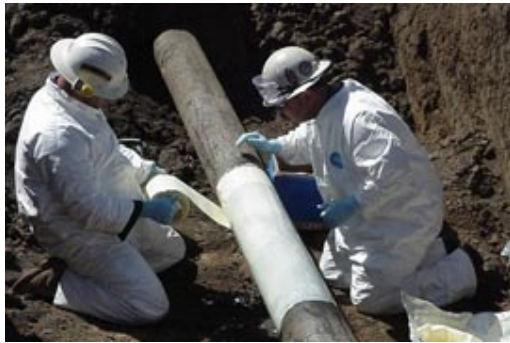
Repair of Corroded Transmission Pipeline
