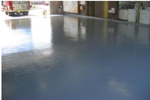
Bridge Deck Sealing (non Skid)
