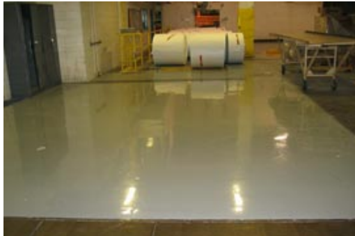
PM Winder Floor After
