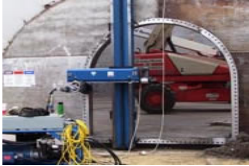
Re-machining access door of tank
