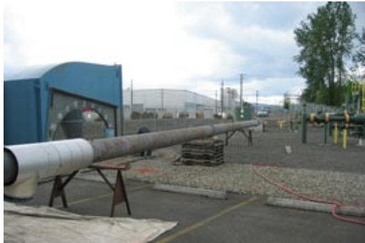
Cogen Stack Before
